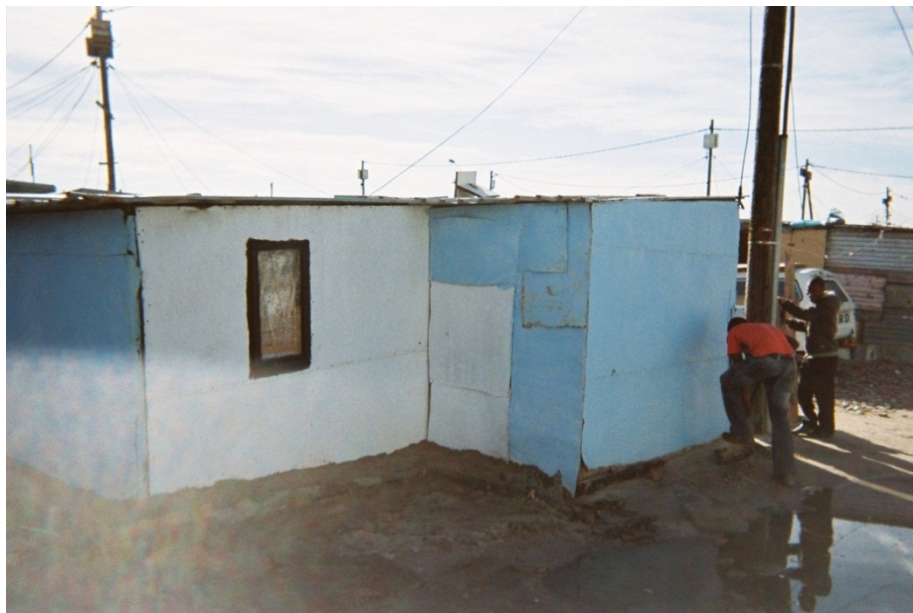
Figure 8: “Here is a place where there was water, so they put cement around the edges of the shack.” (Flooding observer 15.6.2011)
