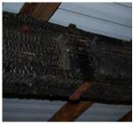
*Figure 88. One of the burnt beams in the roof structure.*
