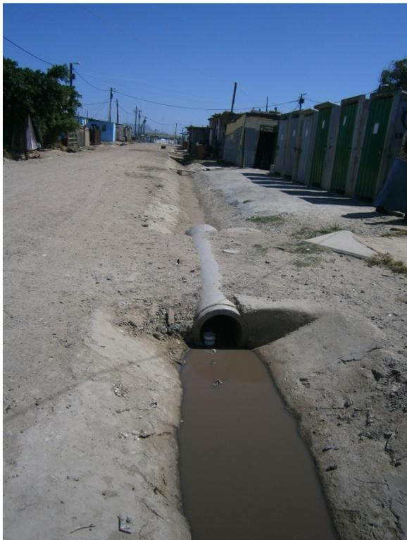
Figure 12: Blocked drain in section G in March (summer season) (Source:Fliccer 2013).
