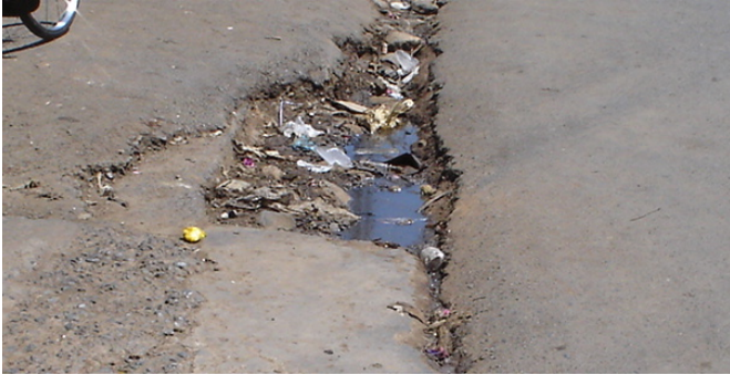
Dumped waste in drains at a Manyatta Mkt.
