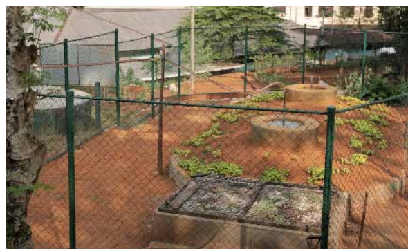
Biogas station at Matale District Hospital - Sri Lanka
