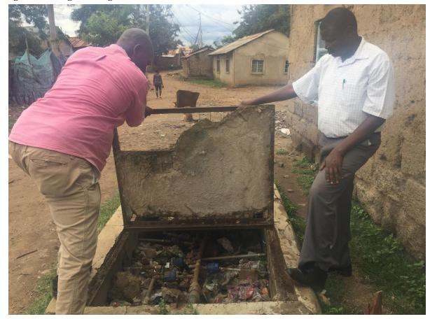
Figure 8.1: Cage holding several DMM water meters
