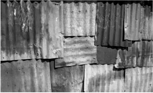
Photo showing a wall made by steel sheets
