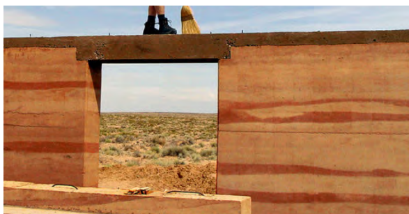
Earth Wall as a thermal mass wall Group 2: What a waste
