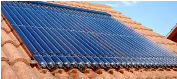
Roof solar panels Group 9: Bråta Recycling Centre
